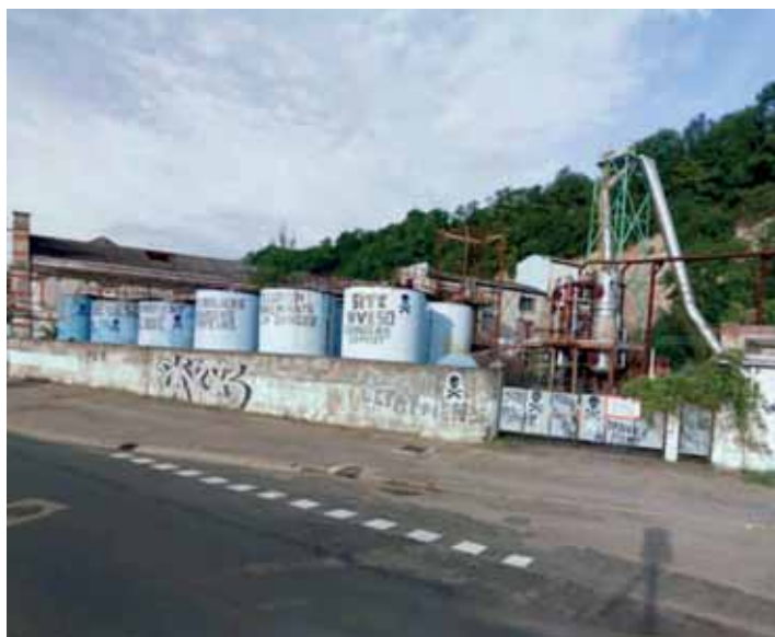
UFP (Petrocarbol) plant in Dieulouard (Meurthe-et-Moselle département)
